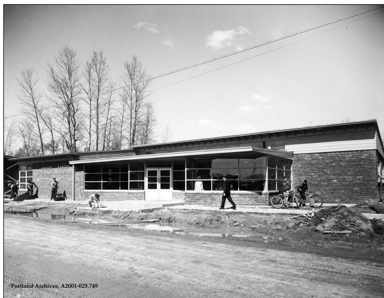
Figure 2. Vanport post office under construction, 1943. Portland City Archives.
