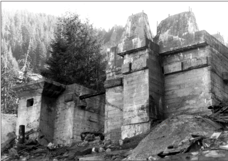
Cement foundations of the Champion mill. Alan Patera photos 1988.
